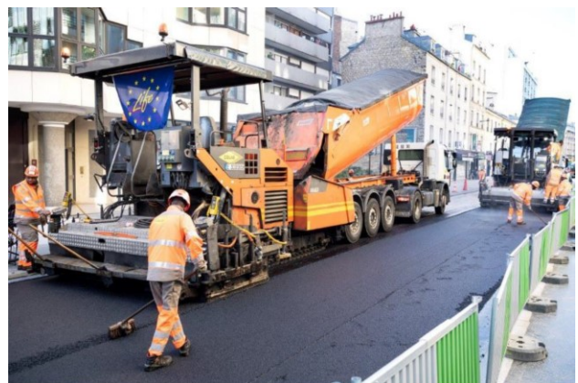
Figure 8. rue Frémicourt with new asphalt mixes, October 2018.
